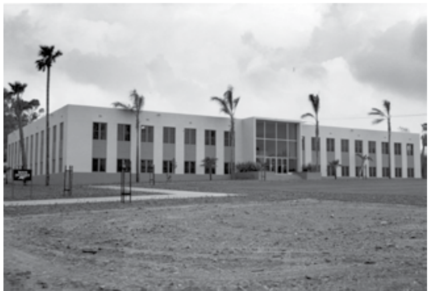
Prince Hall upon completion September 18, 1955
